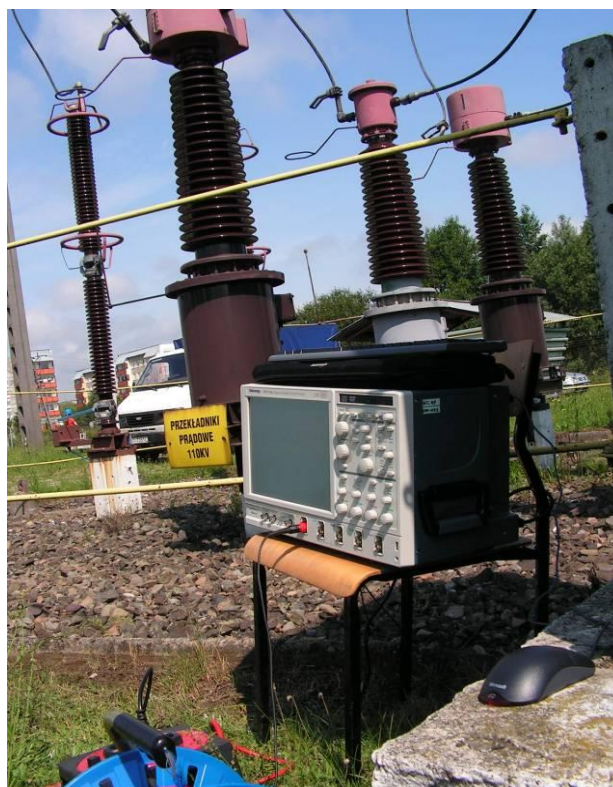
Fig. 1. Ground potential rise measurement process on the high voltage substation
