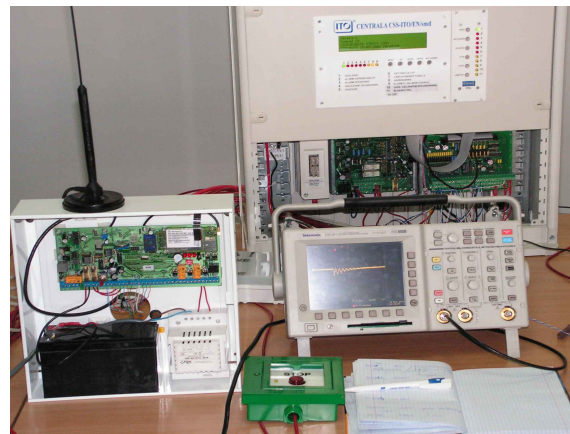
Fig. 1 - Fire protection system during the EMC tests.
