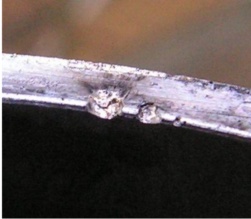
Fig. 4. 8/20 \mu s 1kA surge current result on the flagstaff interconnection point between sections
