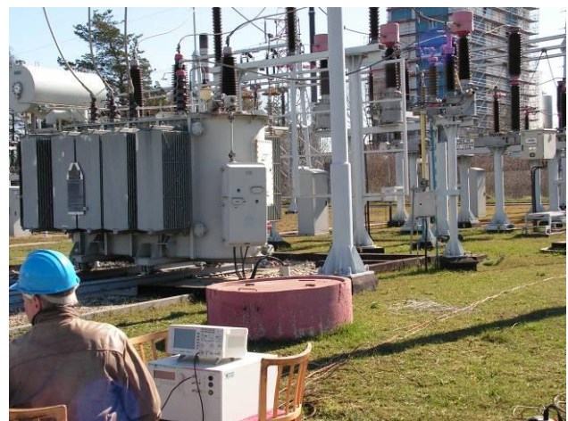
Fig. 1. Ground potential rise measurement process on the high voltage substation
