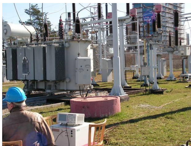
Fig. 1. Ground potential rise measurement process on the high voltage substation
