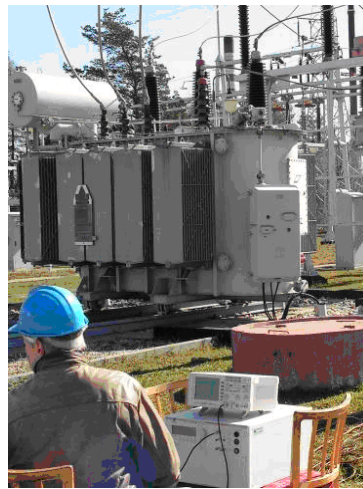
Figure 2. Measurements in progress
